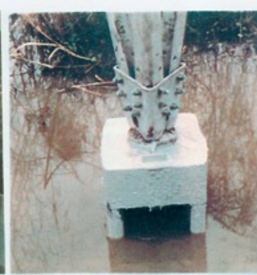
Completed encapsulation of tower foundation.
