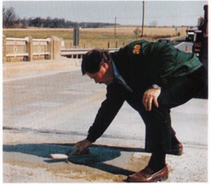
Mr. Carl W. Scheffel, Vice President & Chief Engineer of Fox Industries, checks FX-928 patch before opening lane to traffic. FX-928 achieves 2800 psi in compressive strength in one hour.
