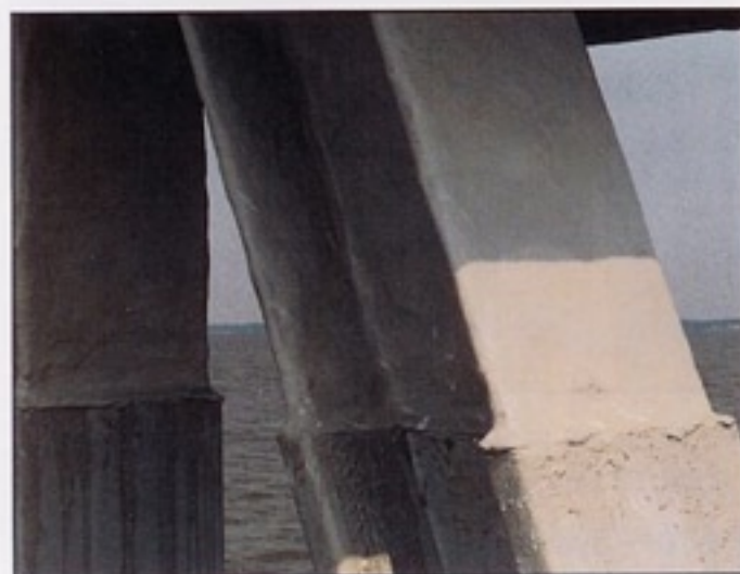
Close-up of completed restoration. FX-763 Trowel Grade Hydro-Ester® Epoxy is applied as a bevel to seal jacket - facilitate run off.
