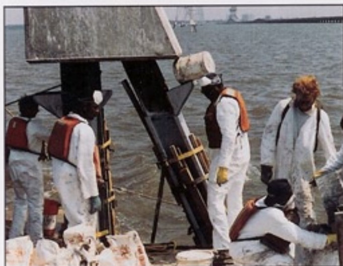
FX-70-6 Hydro-Ester® Pourable Epoxy Grout poured into funnel.
