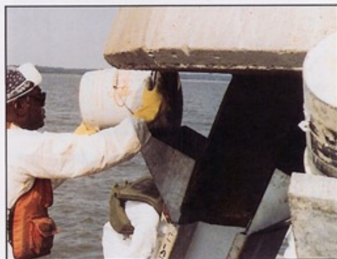
FX-70-6 Hydro-Ester® Pourable Epoxy pours through entrapped water, self levels, consolidates, displaces water and gives tenacious bond.
