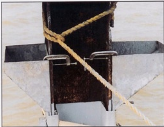
Sheet metal pouring funnels, clamped in place.
