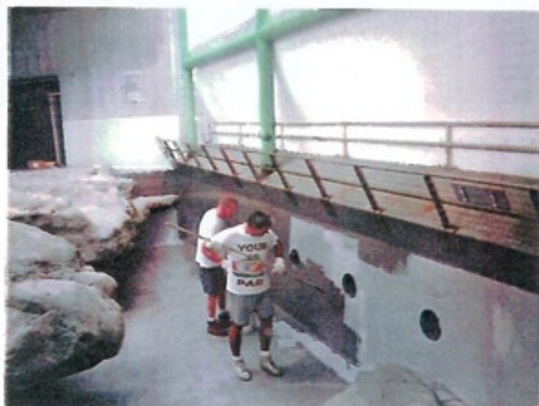
Final layer of inorganic reinforcement is coated with epoxy.
