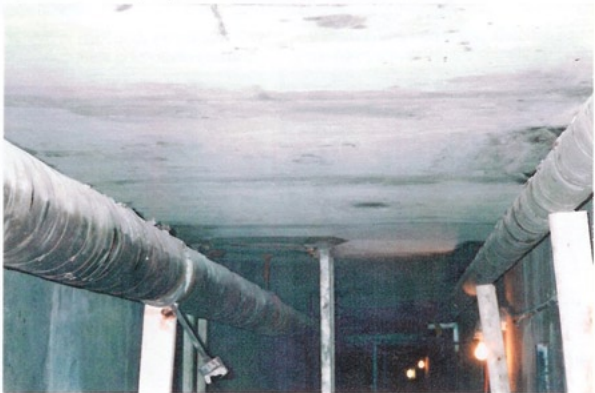
View of completed ceiling section
