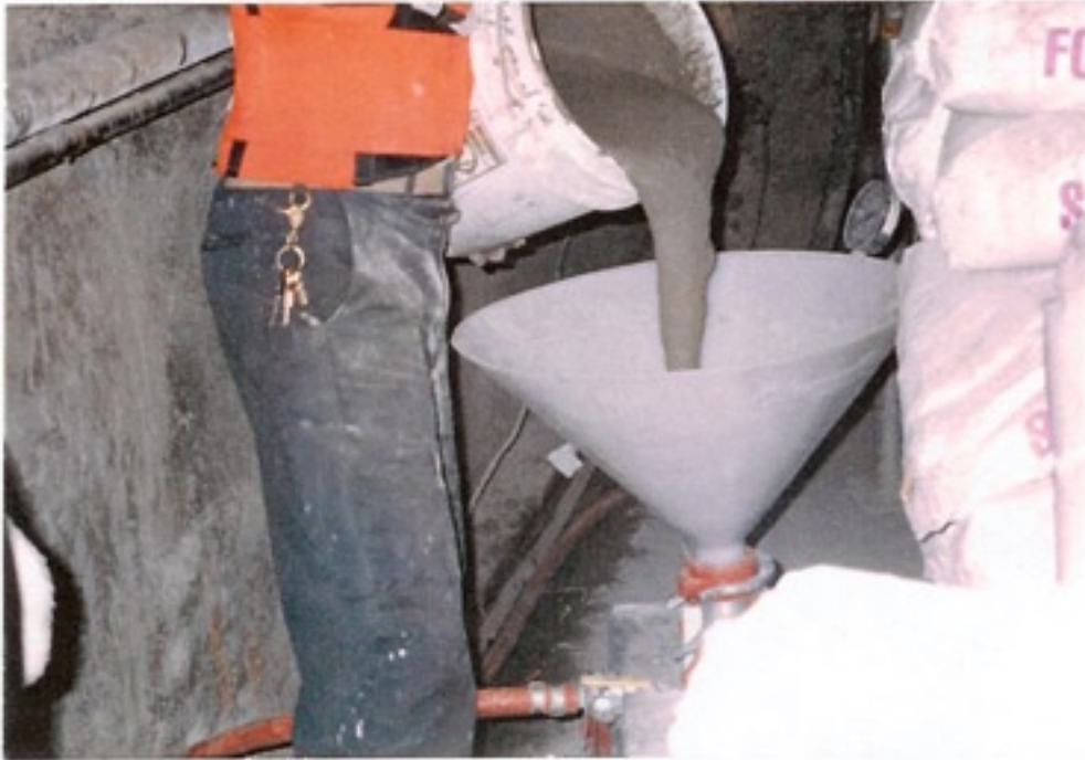
FX-228 Non-Shrink Non-Metallic Grout is easily pumped using an air operated piston pump.
