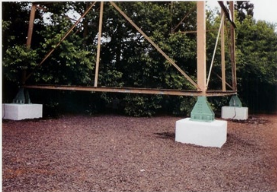
Overall view of completed job.
