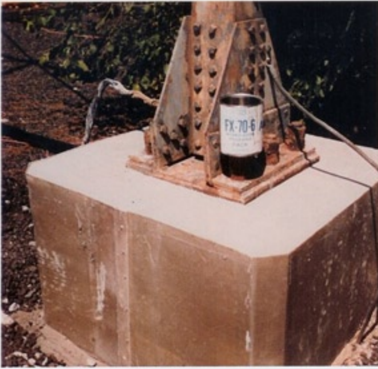
The remaining 2" of void space is filled with FX-70-6 Epoxy Grout .
