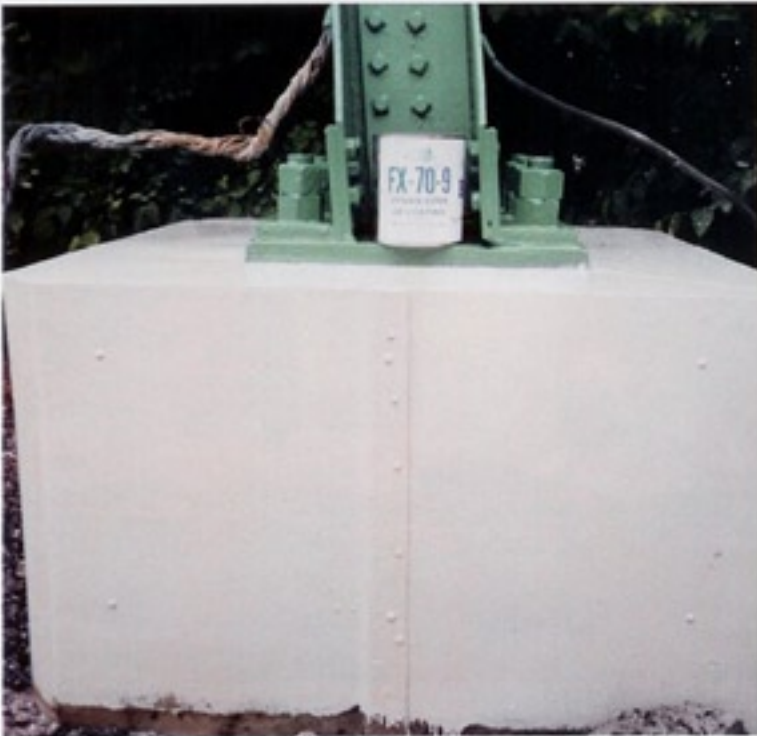
The outside face of the FX-70® Jacket and the FX-70-6 Epoxy Grout are coated with FX-70-9 LV Coating .
