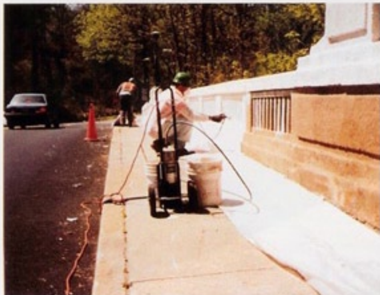
Windsor Mill Road remains open to traffic while FX-460 is applied.
