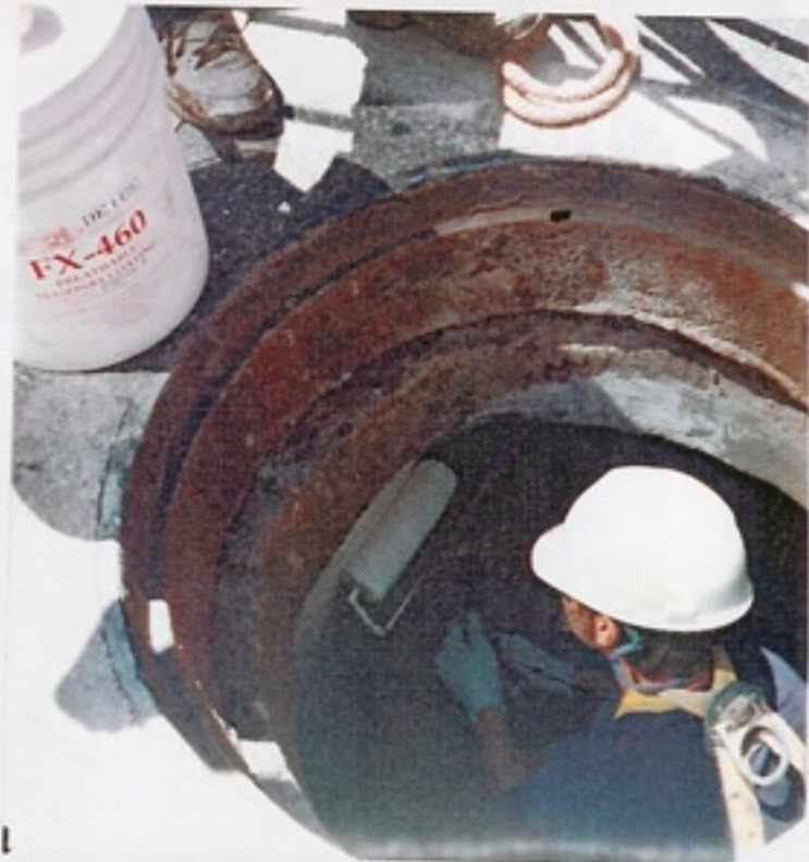
After all patching work has been completed FX-460 Breathable Coating is applied to walls and ceiling of vaults.
