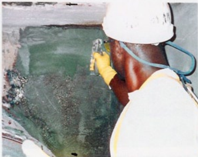
Close up view of technician applying FX-253 Mortar to wall surface.
