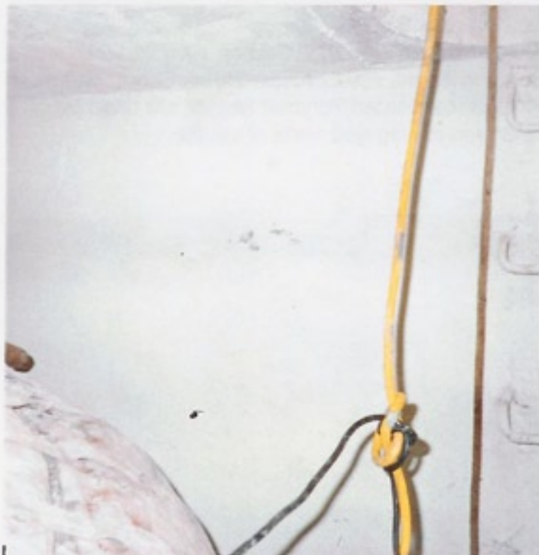
Close up view of completed wall section.
