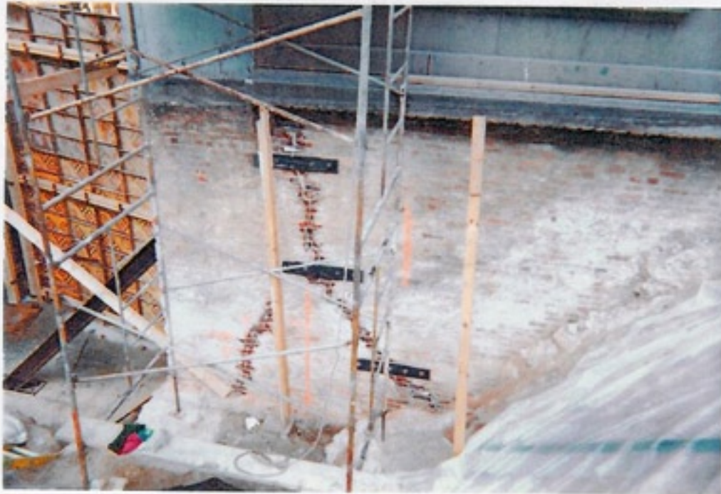
Overall view of completed injection project.
