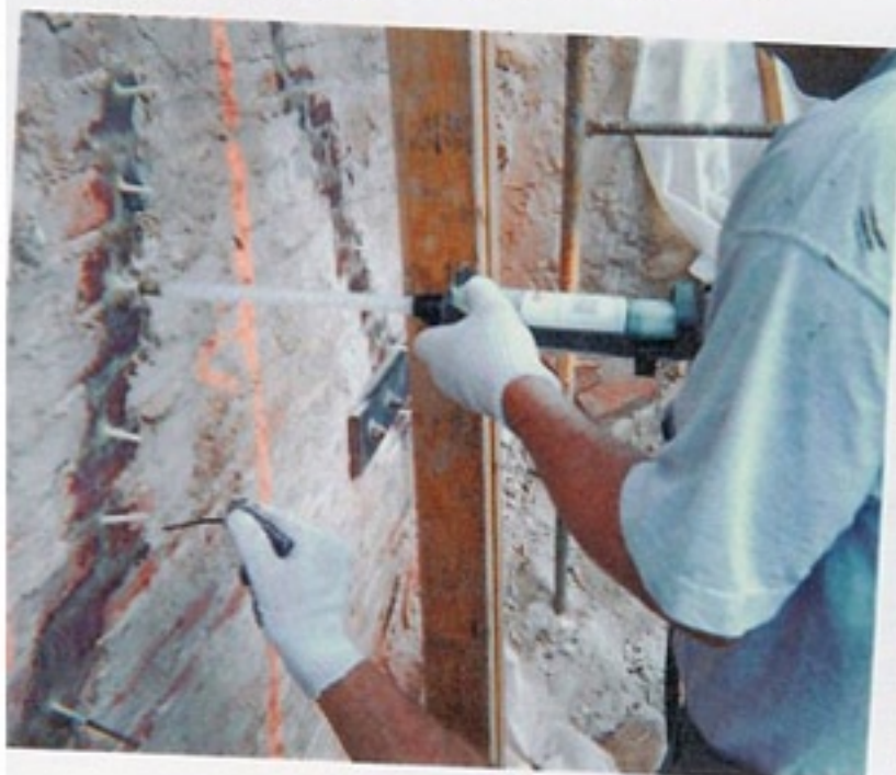
FX-751 LV Epoxy is pumped through ports using air powered handgun and double barrel epoxy tubes with static mixers. (over)
