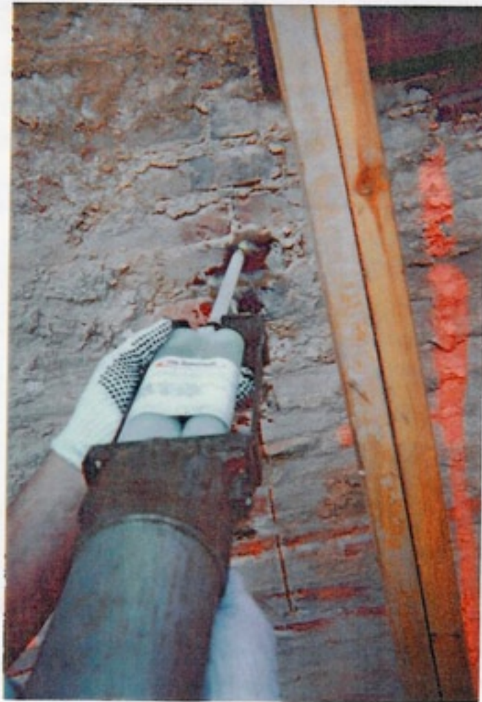
Larger voids are filled with FX-715 Hydro Ester® Non-Sagging Consistency.
