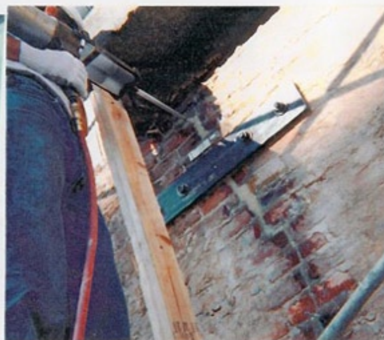
Using the static mixing heads eliminates the need to premix the injection epoxy.
