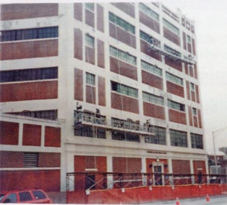
Repairs are being performed using swing stage scaffolding.
