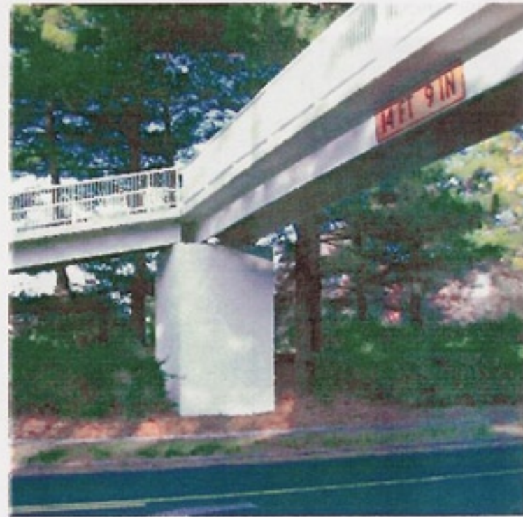
View of completed bridge with new railing and FX-460 Breathable Masonry Coating. The bridge was repaired under strict time constraints allowing students to access their elementary school without crossing dangerous intersection.
