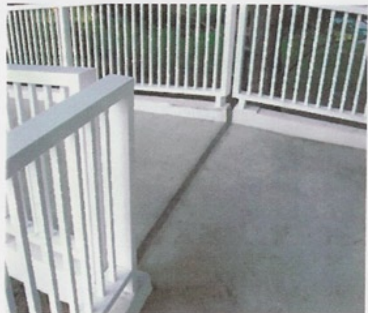
Both sides of joint area were repaired with FX-32 Concrete Mix creating a two inch joint. FX-555 Preformed Sealer was placed in the joint.
