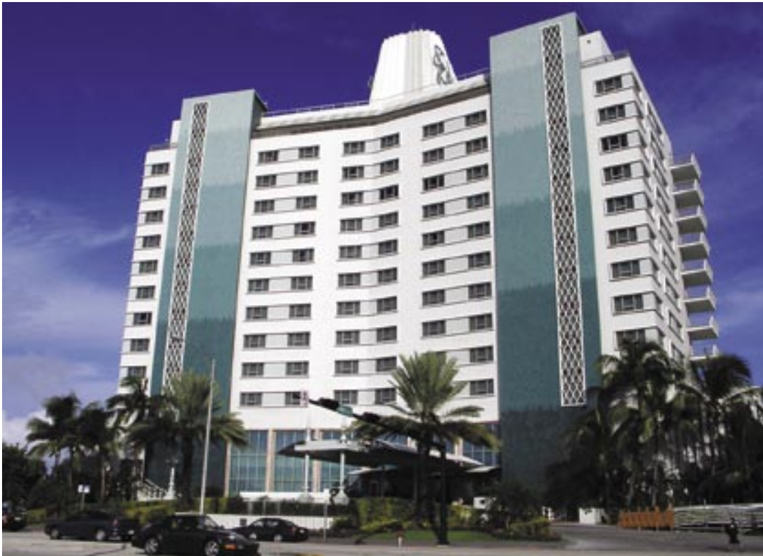
Eden Roc Hotel entrance with its two tiled towers in their full glory
